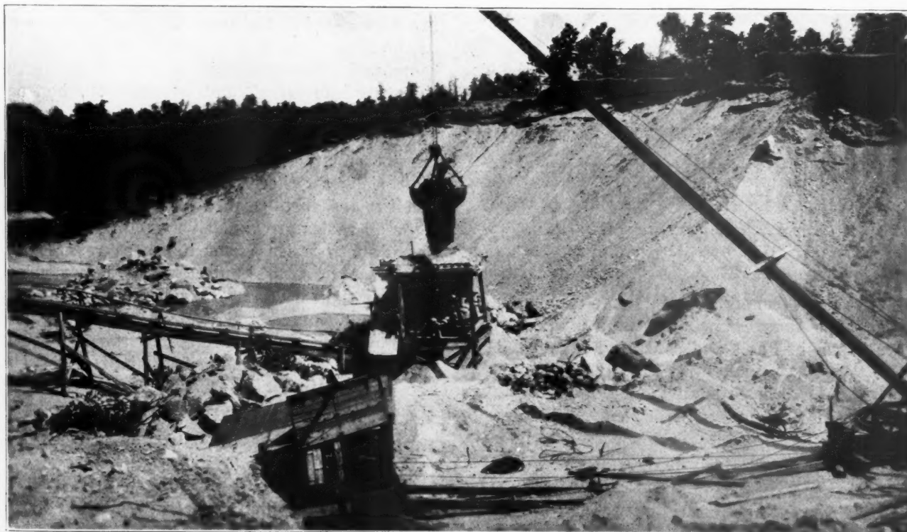
Bucket Dumping into Hopper. Note Water Level indicated by Pools in Left Background
